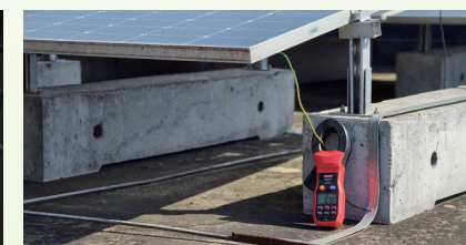
Measurement of Ground Resistance of solar Panels
