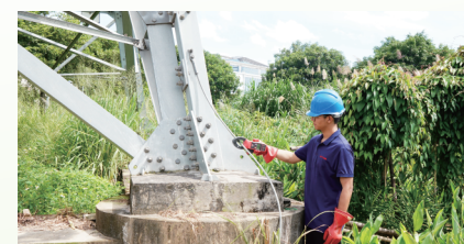
Measurement of Tower Ground Resistance
